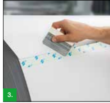
Figure 3: Attach the paper top layer onto the exposed adhesive part of the tape.
