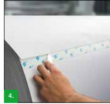
Figure 4: Fold back and remove excess paper tail.
